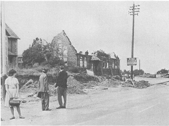
33. The School in demolition, (July 1964).
