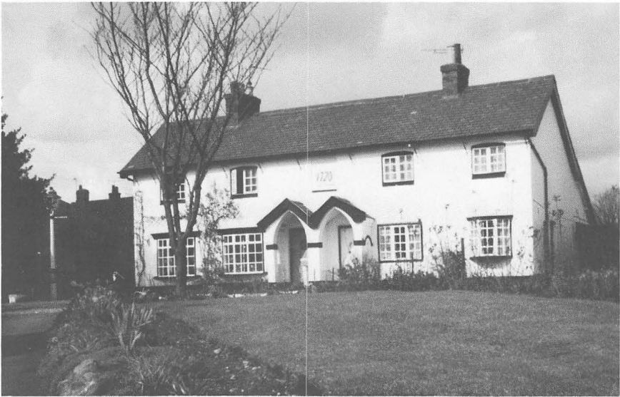
11. Main Street, semi-detached houses. (March 1983).
